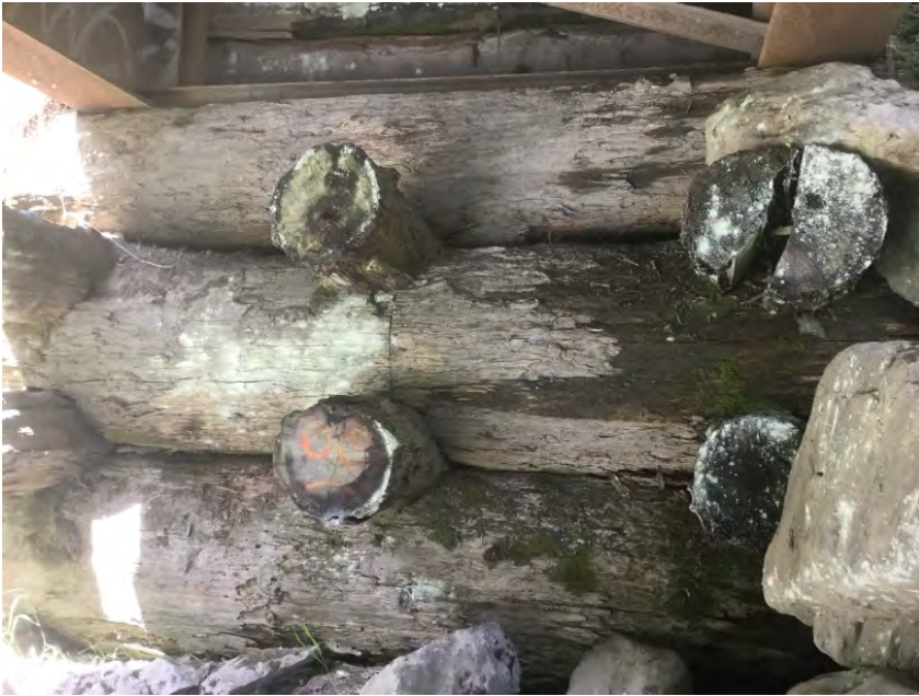
Log crib condition
