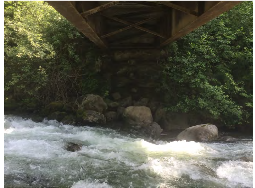
Left Bank Abutment when facing downstream
