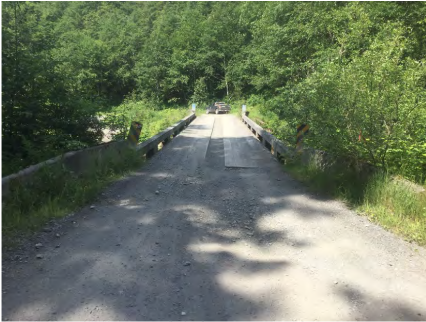
Approach from Left Bank when facing downstream
